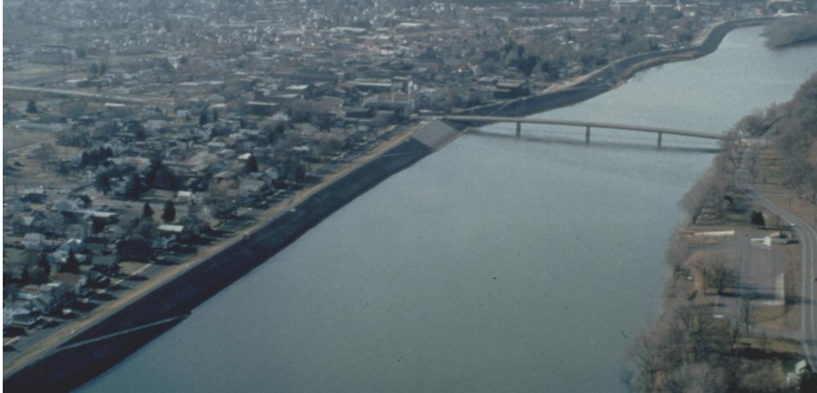
Flood Protection Levee Lock Haven, PA
