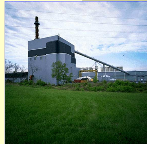
Circulating fluidized bed (CFB) facility at NorthamptonAllentown, Pennsylvania, USA ( www.power-technology.com )
